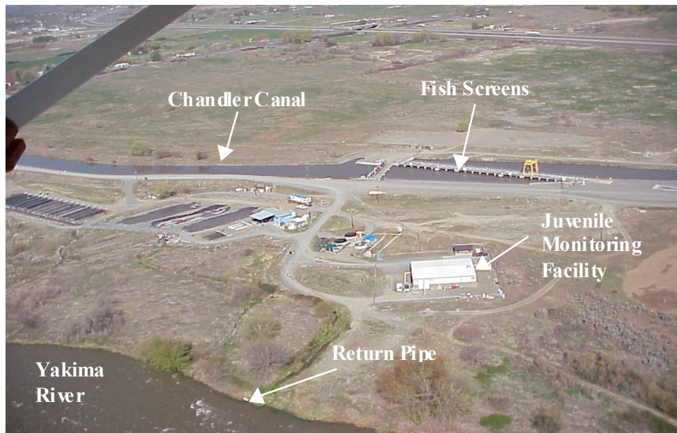
Figure 2.6. Chandler Canal Fish Screen and Juvenile Monitoring Facility on the Yakima River. Photo courtesy of Yakama Nation.
